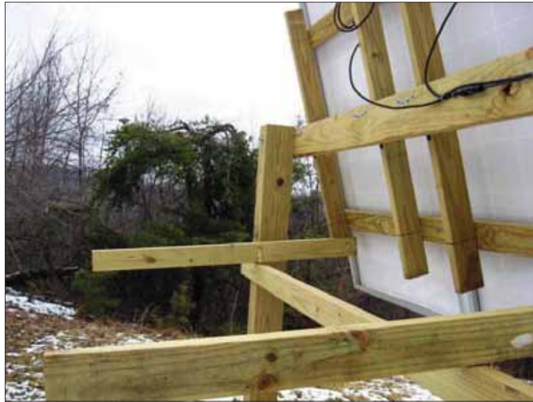
The angle of the solar panels is changed by moving the horizontal boards pictured in this photo forward, tilting the bottom of the panels upward at an angle toward the higher spring and summer sun. photo by Mary Wildfire
