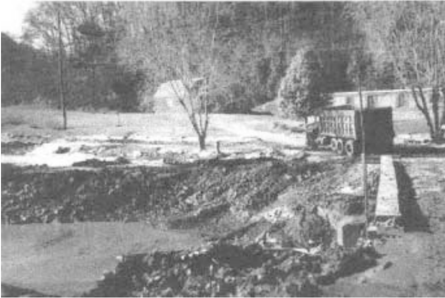
A large dump truck hauls away a tiny portion of the coal slurry from Coldwater Creek. The bridge at right had been completely covered by the goop.
