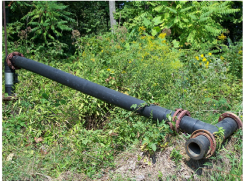
“Coal Slurry Injection Site”
