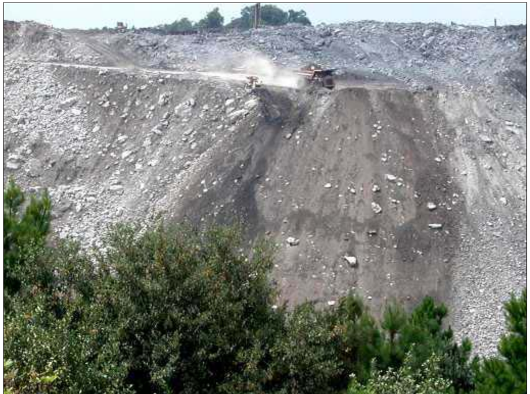
Giant bulldozers and dump trucks are dwarfed by the scale of destruction that is mountaintop removal mining in Mingo County, WV.
