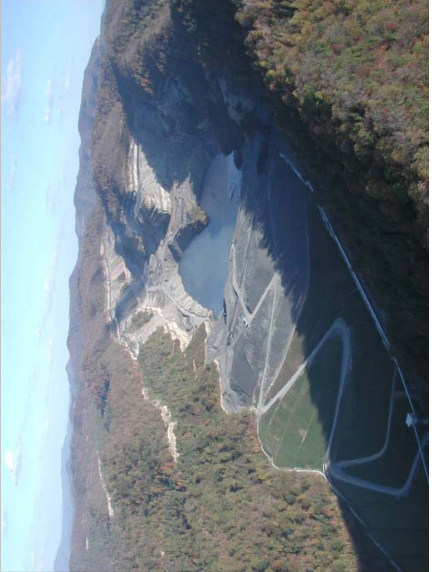
Marfork Coal Co.'s (Massey Energy) massive Brushy Fork impoundment near Whitesville, WV, is designed to hold 8 BILLION gallons of sludge.
