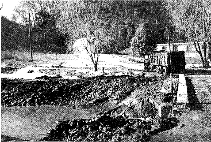
A large dump truck hauls away a tiny portion of the coal slurry from Coldwater Creek. The bridge at right had been completely covered by the goop.
